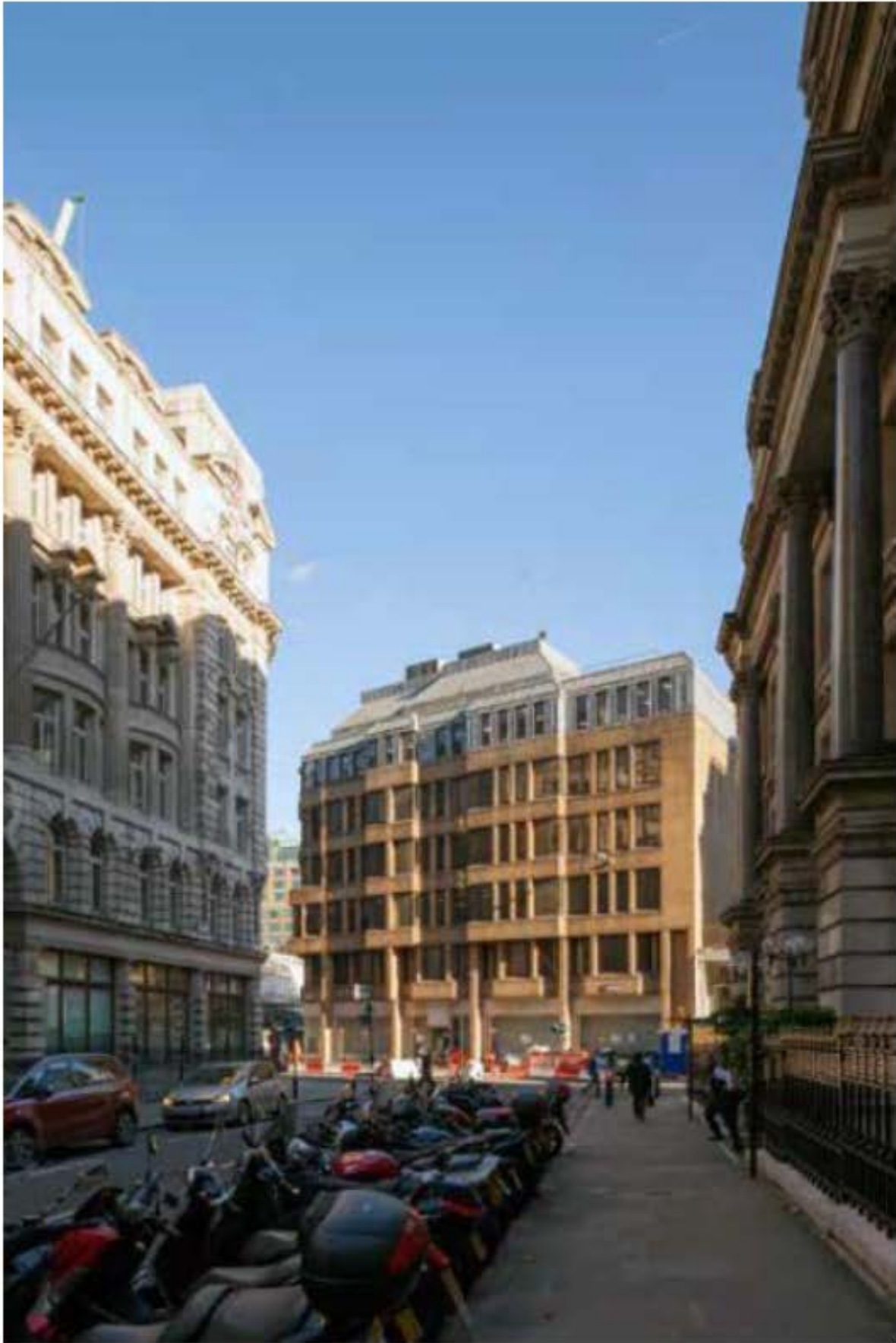
View of the site looking east from Finsbury Circus
