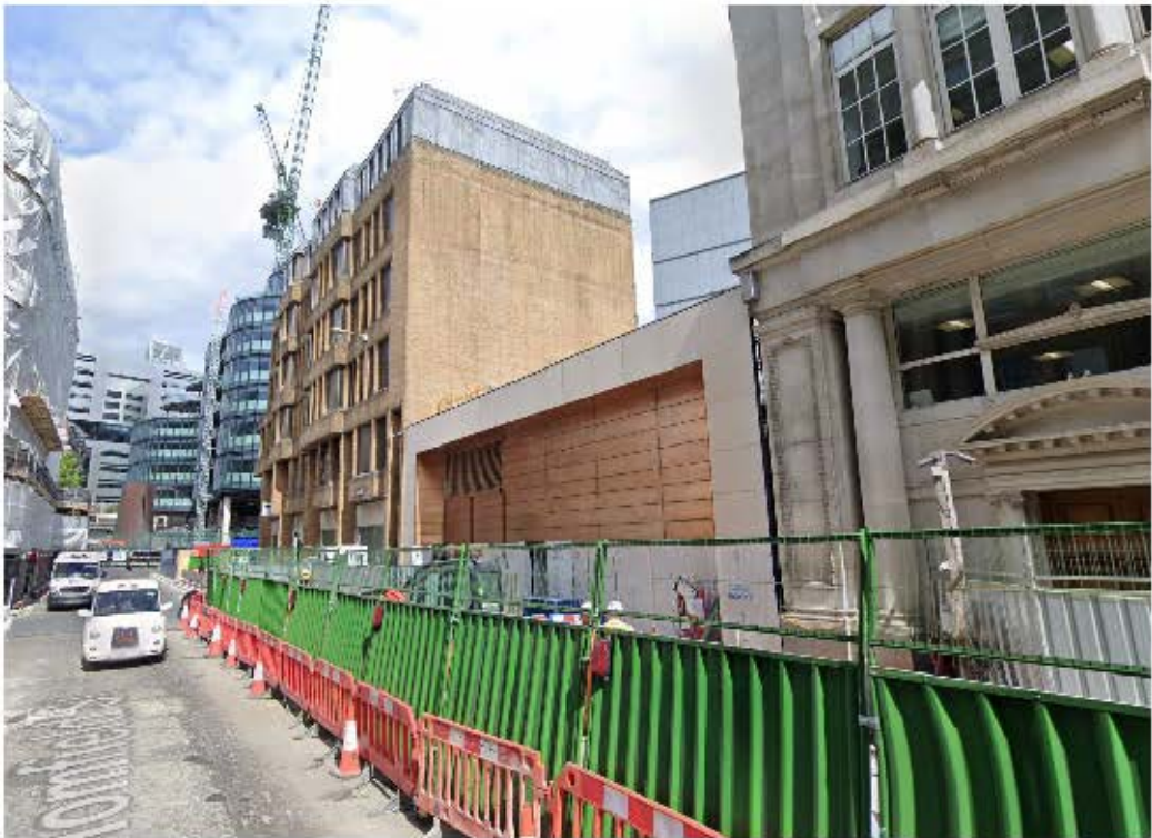
View of the site looking north along Blomfield Street
